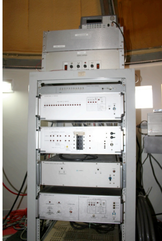
Figura 2: Rack de drives
