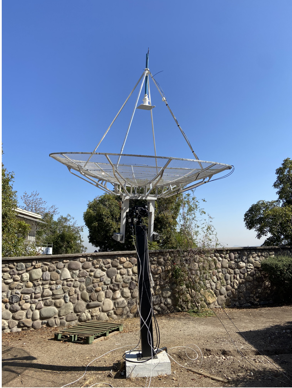
Figure 5.1: Photograph of the CPT project featuring a single-ended LNA installed at Cerro Calán, Chile. The LNA is mounted connected to the antenna at the feed using a custom 3D-printed support structure, ensuring optimal placement and stability. This implementation demonstrates the practical application of the single-ended LNA and serves as a precursor for the larger-scale CHARTS array.
